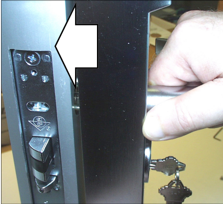
Fig. 6: Install lock onto the door
