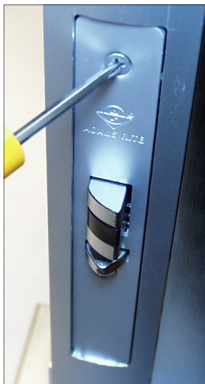
Fig. 5e: Install the latch face plate
